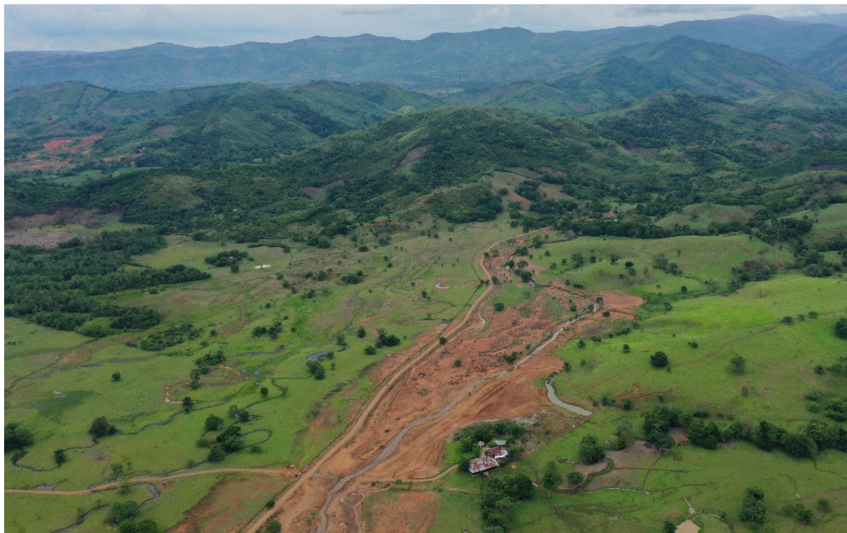
The Valdez stream and flood Plain running through the historical tailings area.
